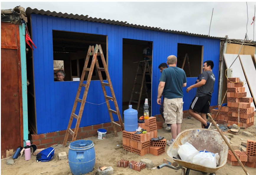
Nearing completion on the new house!
